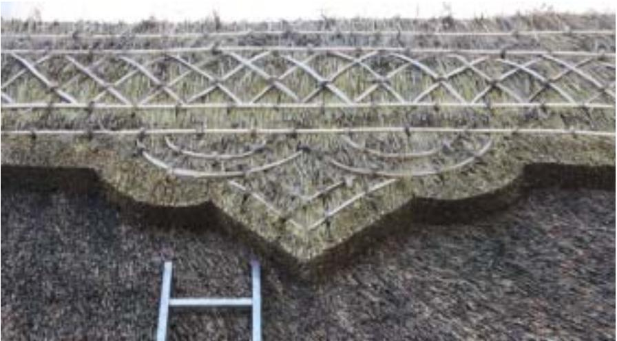
The main part of the thatch was also scraped off to remove accumulated moss and debris, and re-dressed with a leggett to form neat edges. Finally the ridge was covered in galvanised wire netting, to improve durability (the wind howls across Old Hall Field), and to prevent birds from removing all the new straw for nest material !
